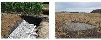
The blind inlet shown above was constructed with about 15 tons of steel slag which removed over 45% of the 3-yr DP load, plus >70% of glyphosate and dicamba. Note that blind inlets constructed with the traditional imestone material will not remove DP due to low calcium solubility.
