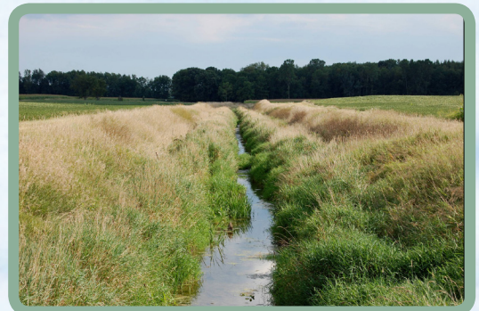
Figure 1. A two-stage channel system 6 years after construction.
