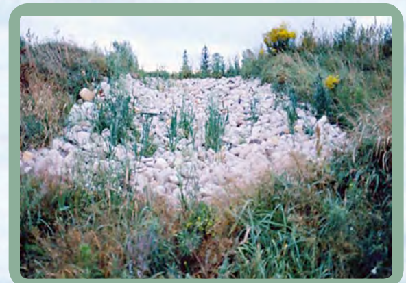
Figure 11. Rock chutes concentrate runoff from fields and direct it into the ditch. (source: http://www.omafra.gov.on.ca/english/engineer/ )
