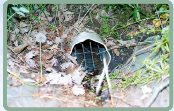
Figure 6. Animal guards on the end of a subsurface tile help prevent damage and clogging. (source: http://www.ipm.iastate.edu/ )
