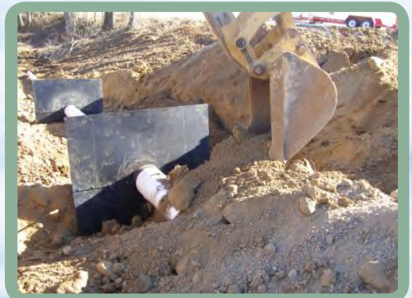
Figure 7. Anti-seep collars installed on a subsurface drainage project. (source: http://swcd.mo.gov/drainage.html )
