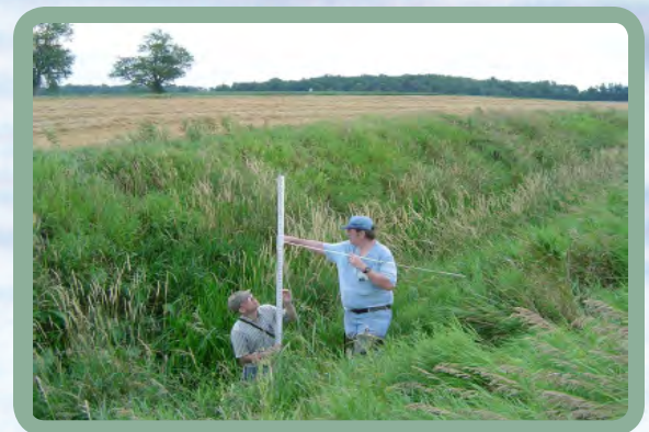
Figure 13. An engineering survey of an existing trapezoidal channel prior to two-stage construction.
