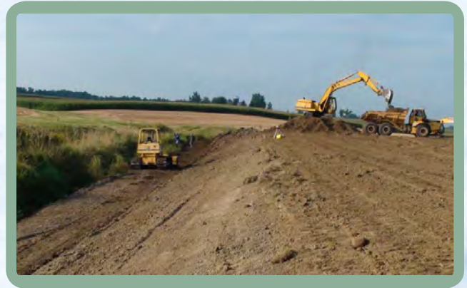
Figure 4. Excavation and grading on a two-stage channel project.
