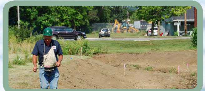
Figure 9. Site seeding using the broadcast seeding method.
