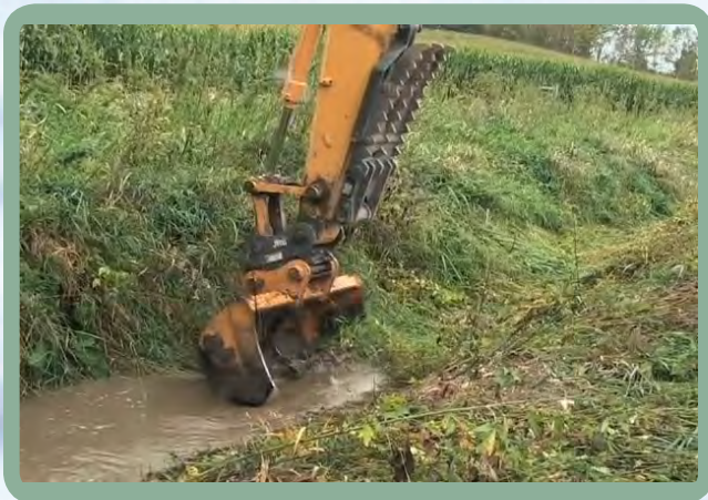
Figure 3. Removal of sediments on the channel bed during a traditional clean-out.
